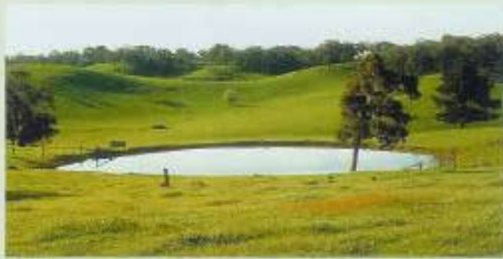
A shallow farm dam can lose up to 40 per cent of its water annually to evaporation. (Graham Strachan)
